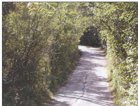
A property's landscaping may not offer enough clearance for emergency vehicles.
