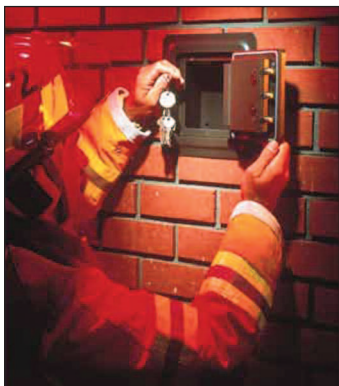
A Knox-Box lets emergency personnel access a property without using force.
